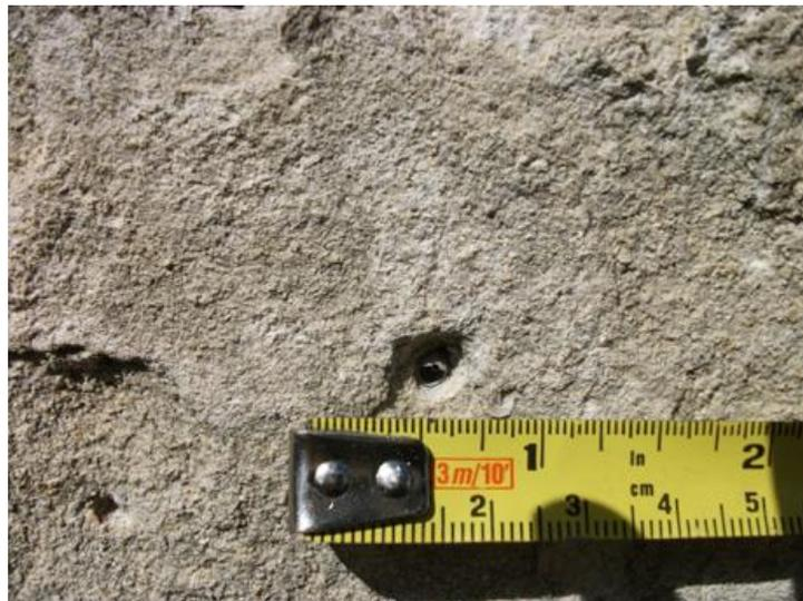
Fig 1a: Enlarged pits visible on the border wall at the University of Oxford Botanic Garden
