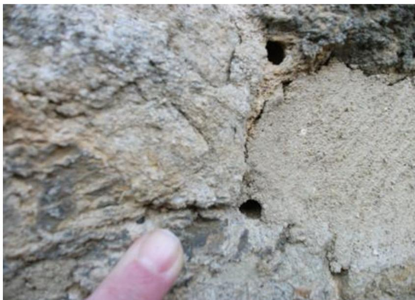
Fig IVb: Similar pitting observed on a different wall (belonging to Merton College, Oxford) known to be occupied by bees, with boring preference near to mortar
